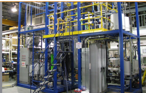
19 L 8-zone furnace packed bed
